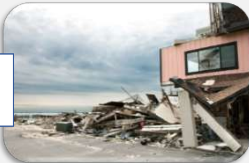
Damage caused by a hurricane.
